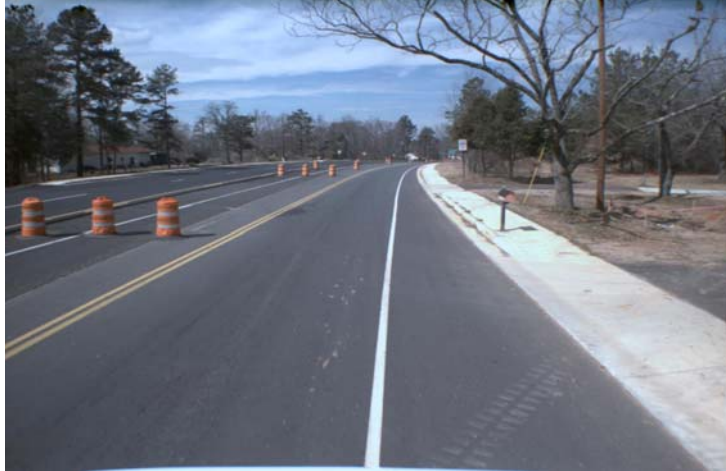
Figure 5 Site identified as having recent reconstruction using video-log
